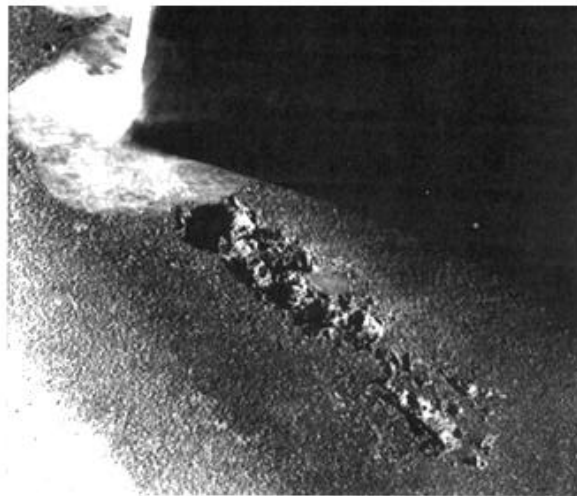
Figure 5. Cavitation Pitting in Turbine Blade (Source: Jones, pg. 349)
