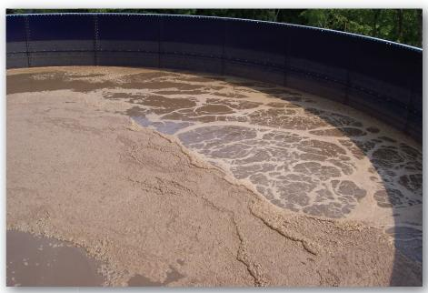
This design using Rotamix with Air in 5% solids resulted in only two required digesters versus three required using standard aeration technologies. Blower capacities were reduced from 30-35 SCFM to less than 15 SCFM while maintaining 3mg/l of dissolved Oxygen.
